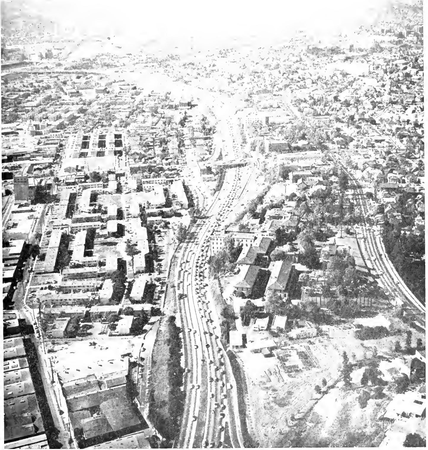
Looking northerly along Santa Ana Freeway in East Los Angeles area from above Sixth Street, showing Fourth Street Overcrossing in center
